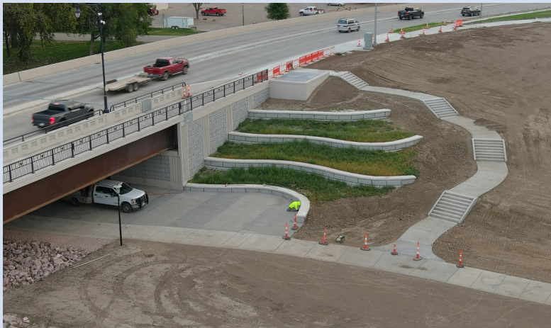
Retaining wall and stair installation on the Pierre side plaza area. (Oct. 2025)
