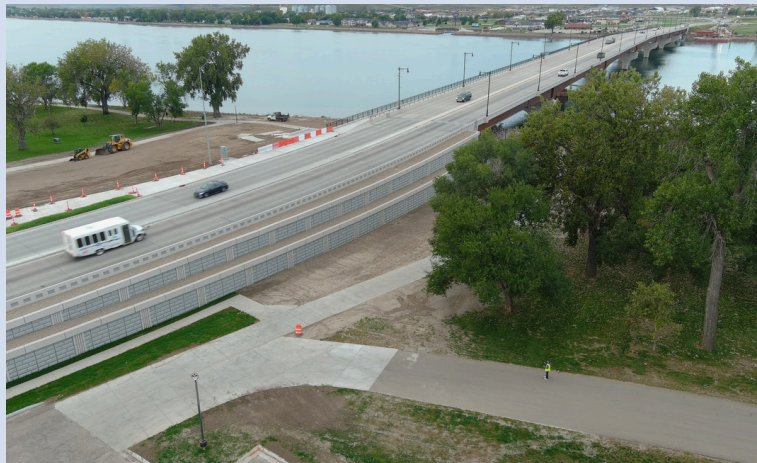
Retaining wall and stair installation on the Pierre side plaza area. (Oct. 2025)
