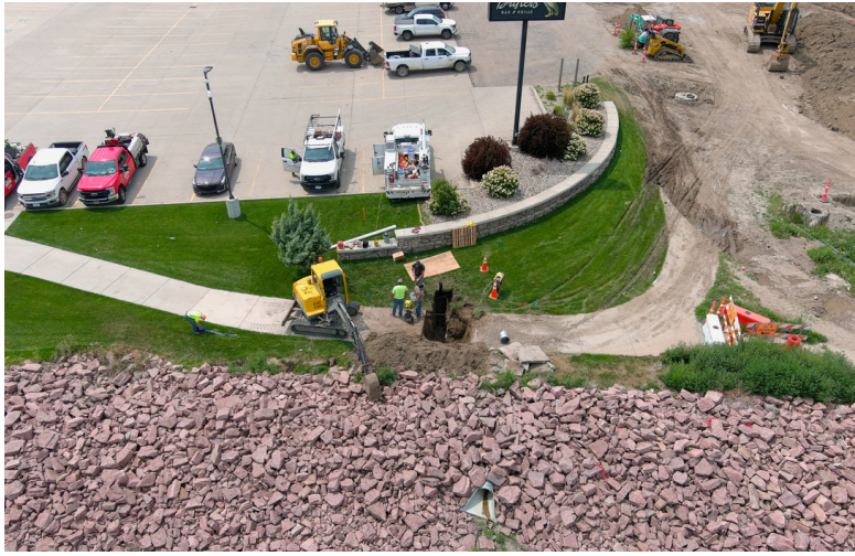
Riprap placement and plaza work on the Fort Pierre side. (July 2025)
