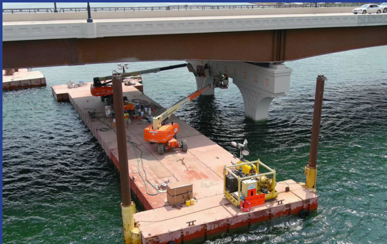
Progress continues on the water as well. Painting and concrete footing removal continue. (July 2025)
