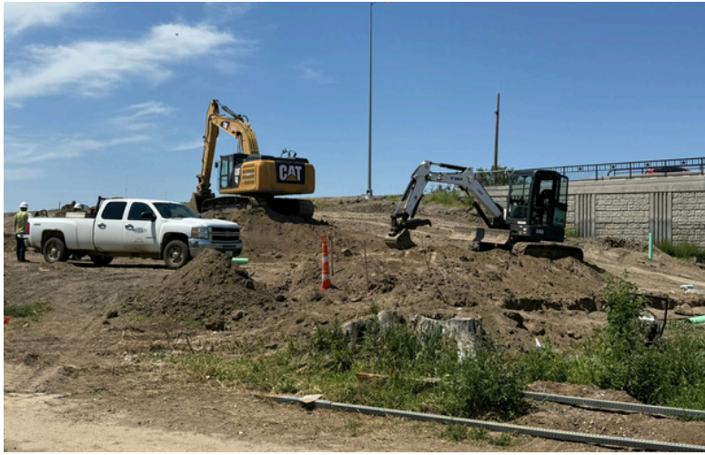
Grading work continues for the stairway and block retaining wall on the Ft. Pierre side. (July 2025)
