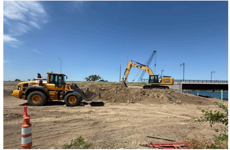
Grading work continues for the stairway and block retaining wall on the Ft. Pierre side. (July 2025)
