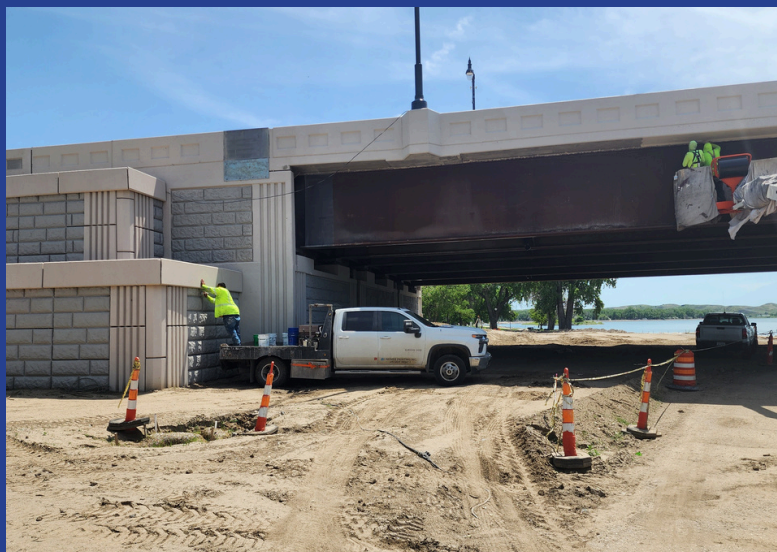
Crews are working on painting the new bridge. (June 2025)
