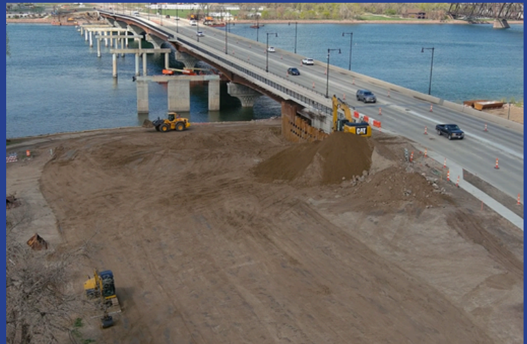
Grading and excavation work continue as part of the plaza development on the Pierre side of the bridge. (May 2025)
