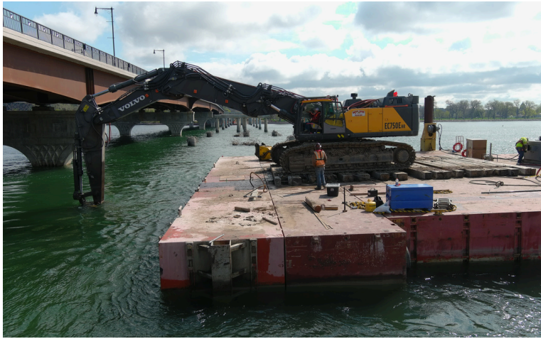
Crews have begun demolition of the existing bridge piers which will continue through the summer. (May 2025)
