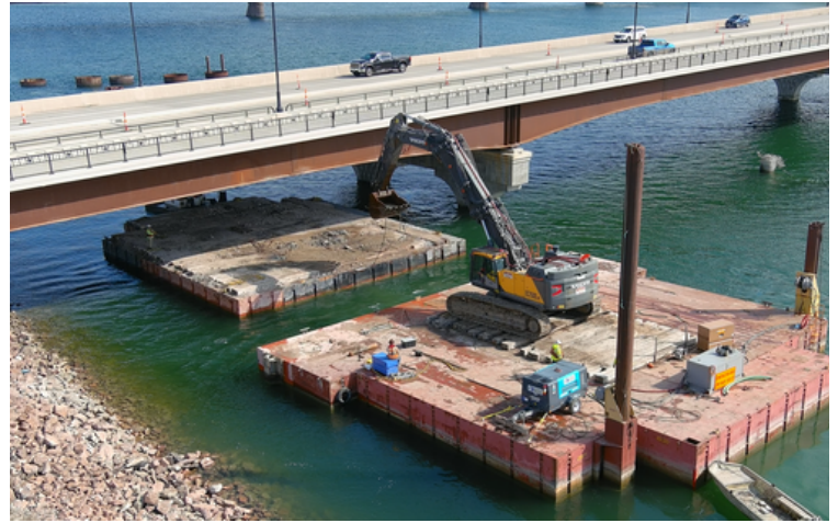
Crews have begun demolition of the existing bridge piers which will continue through the summer. (May 2025)
