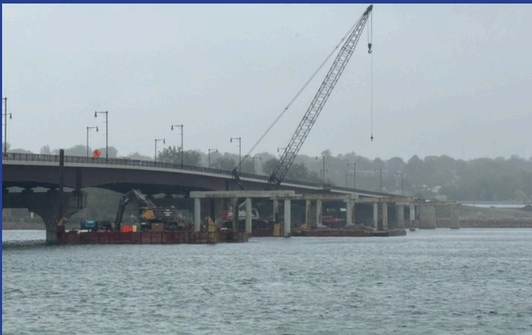
Despite rainy conditions, crews continue demolition of the existing bridge piers. (May 2025)
