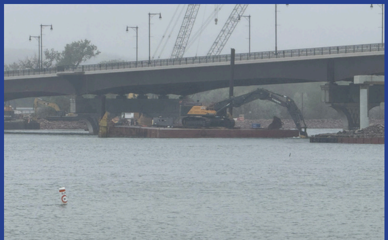
Despite rainy conditions, crews continue demolition of the existing bridge piers. (May 2025)
