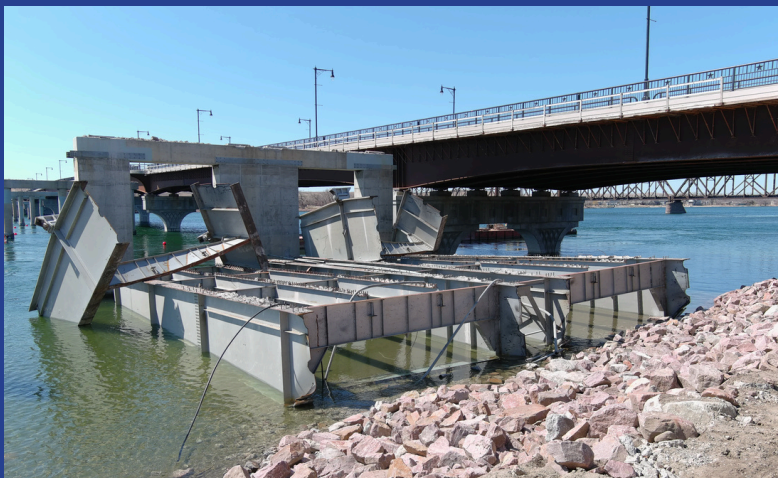
Steel from the girder demolition is disassembled, removed from the river, and stored on site until it is hauled away. (Apr. 2025)
