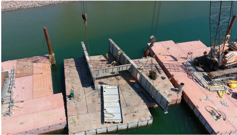
Crews continue pulling debris from the girder demolition out of the river. (Apr. 2025)
