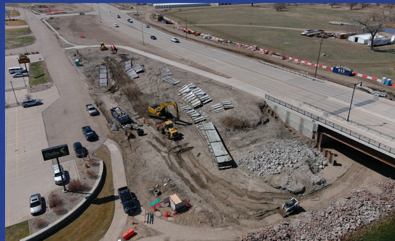
Steel from the girder demolition is disassembled, removed from the river, and stored on site until it is hauled away. (Apr. 2025)
