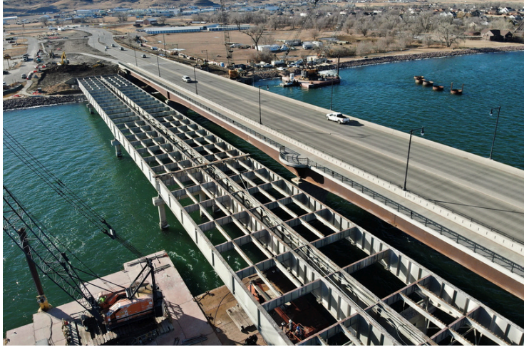
Removal of intermediate steel pieces from the old structure. (Jan. 2025).
