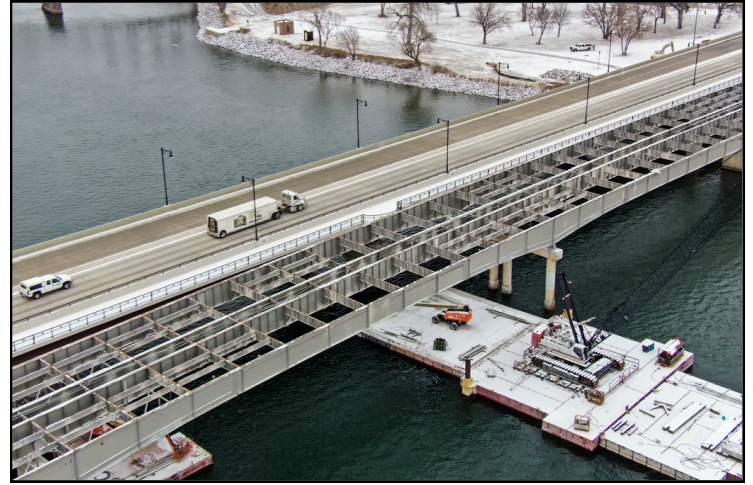
Removal of steel supports from existing bridge on Jan. 14, 2025.
