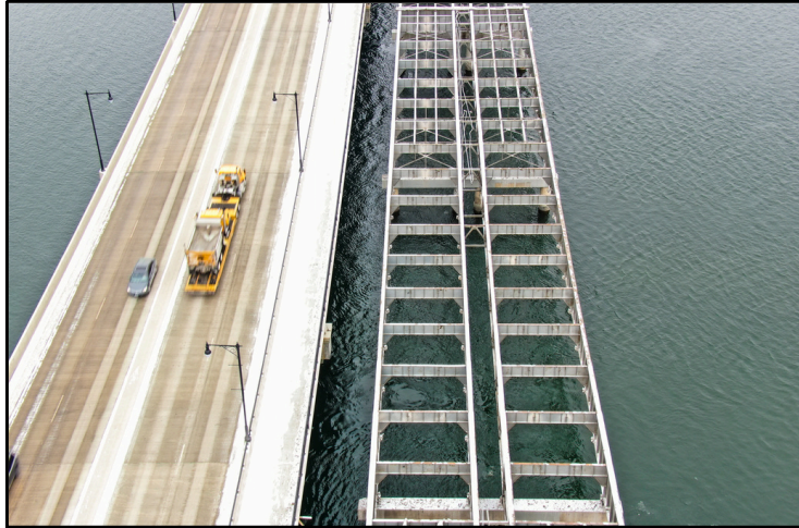
Removal of steel supports from existing bridge on Jan. 14, 2025.
