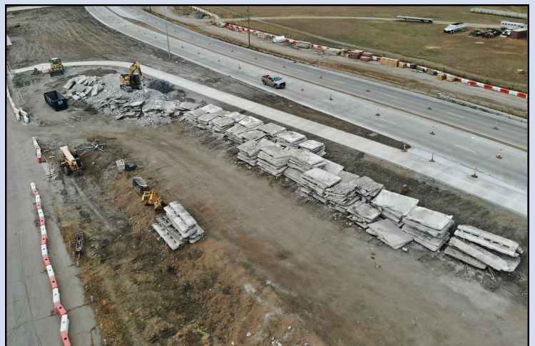
Slabs from existing bridge deck removal. Dec. 2, 2024.
