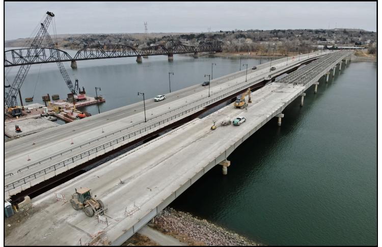
Bridge deck removal status from Ft. Pierre. Dec. 2, 2024.
