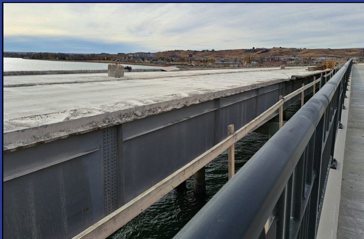
Bridge deck removal. Nov. 18, 2024.
