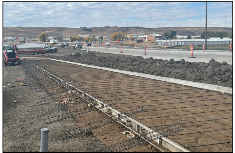
Forms for concrete placement on Fort Pierre-side. Oct. 22, 2024.
