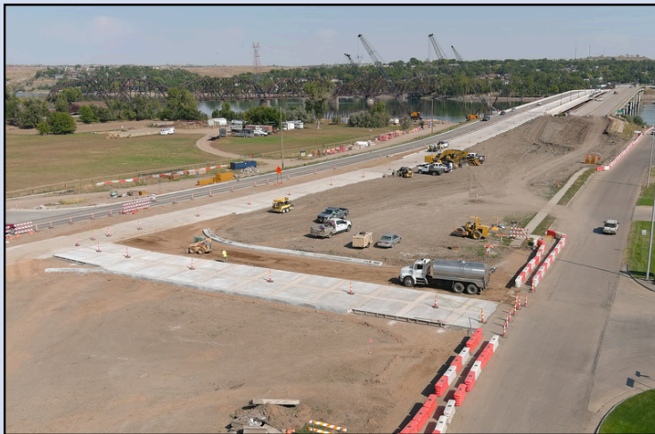
Concrete, curb, and gutter work on Island Drive. Oct. 7, 2024.
