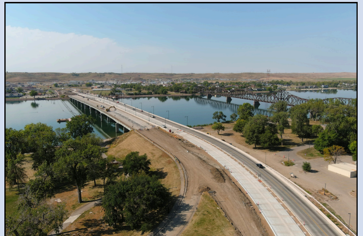
Pierre-side approach and old lane removal. Oct. 7, 2024.
