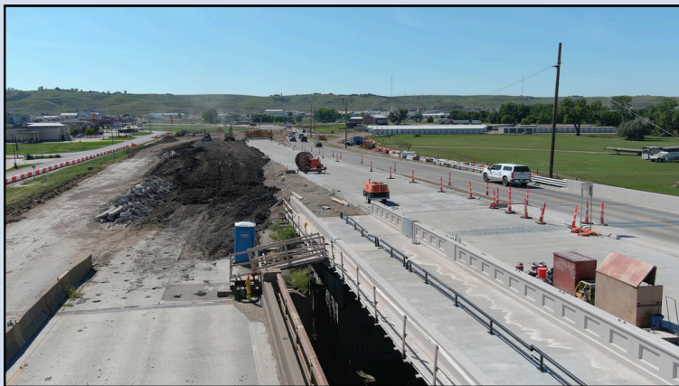
Concrete demolition, earthwork, and the new pedestrian pathway on the Ft. Pierre side. Sept. 6, 2024.
