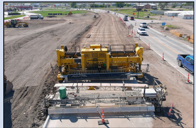
An automatic concrete roller paver places eastbound approach slab on the Ft. Pierre side. Sept. 6, 2024.
