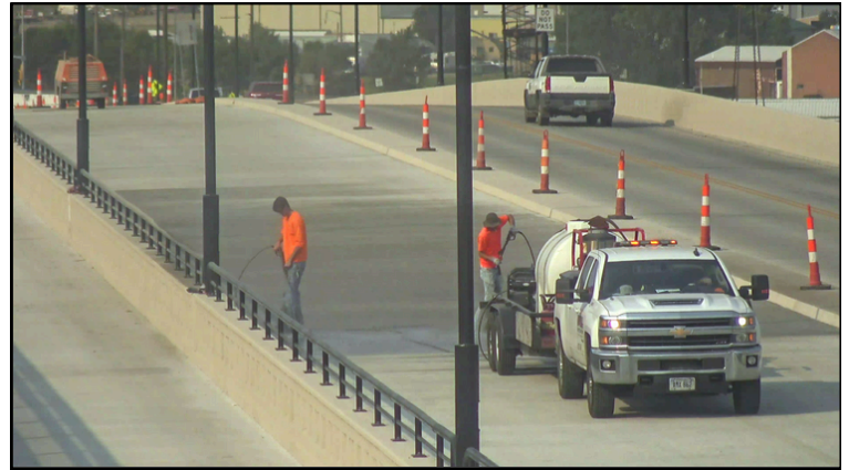
Workers power wash the new deck concrete in preparation for upcoming deck sealant. Sept. 10, 2024.
