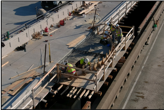
Workers place rebar in concrete forms for upcoming belvedere placement. Sept. 6, 2024.
