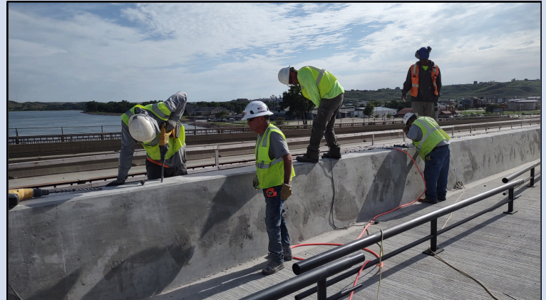
Workers drill holes in the concrete pedestrian separation rail for handrail placement, Aug. 26, 2024.
