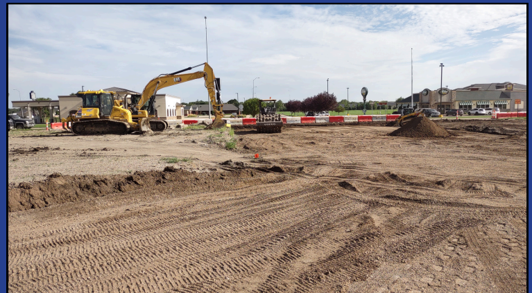
A bulldozer, excavator, and sheepsfoot roller at work on the Island Drive reconfiguration, Aug. 26, 2024.
