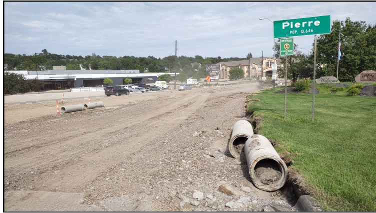
Storm sewer pipe staged on the recently removed approach of the existing bridge on the Pierre side, Aug. 26, 2024.
