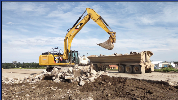
An excavator loads concrete rubble from demolished approach on the Ft. Pierre side, Aug. 26, 2024.
