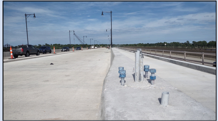
The final luminaire pole awaits installation on the pedestrian separation rail, Aug. 26, 2024.
