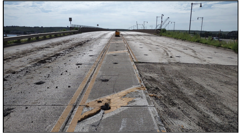
Hydraulic hammer holes and recently removed concrete on the Pierre side of the existing bridge, Aug. 26, 2024.
