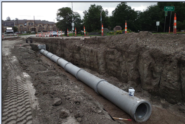
Reinforced concrete pipe in place for upcoming storm sewer work on the Pierre side, July 1, 2024.
