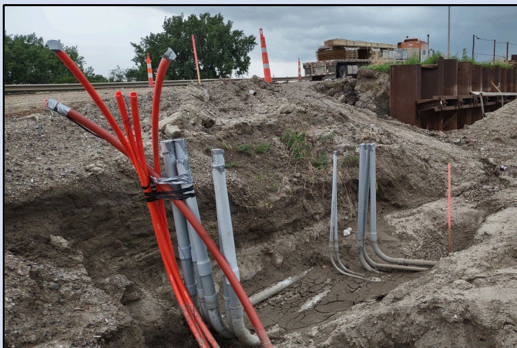
Telecommunications conduit in place for upcoming electrical work on the Pierre side, July 1, 2024.
