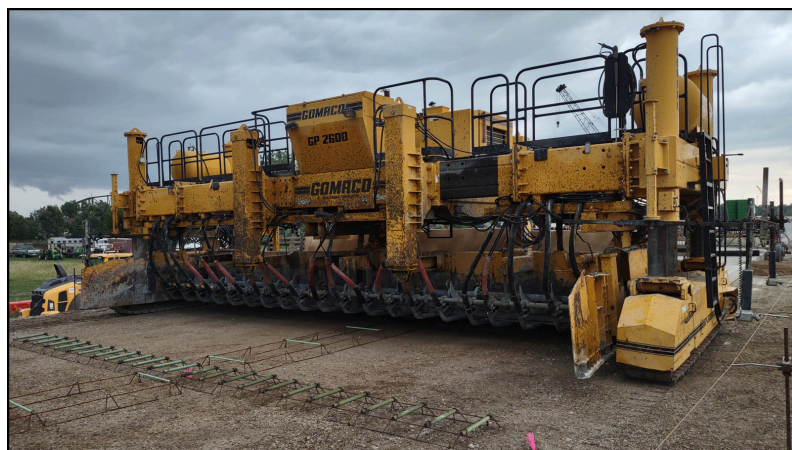
Road paving machine used to place concrete slab on the Ft. Pierre approach (2), July 1, 2024.
