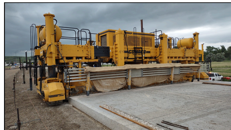
Road paving machine used to place concrete slab on the Ft. Pierre approach (1), July 1, 2024.
