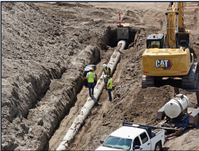
Workers install reinforced concrete pipe for storm sewer, July 15, 2024.
