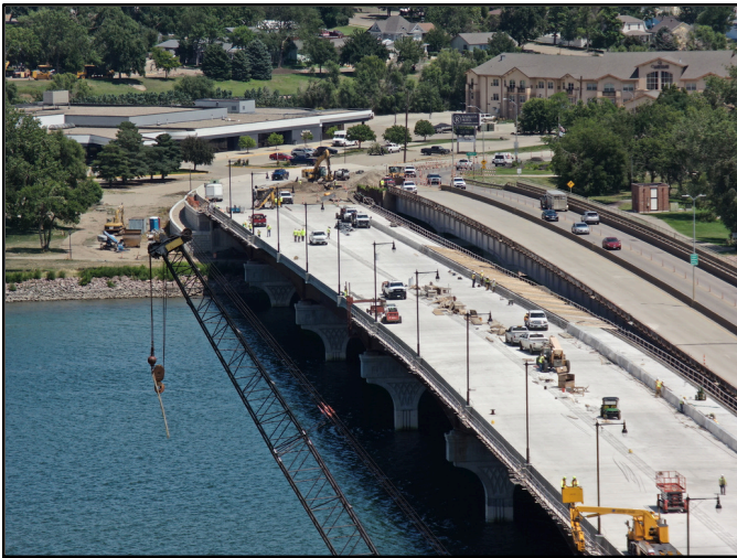
Raised median preparations on the bridge deck, July 15, 2024.
