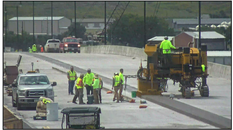
A crew collaborates on raised median placement with the slipform paver, July 16, 2024.
