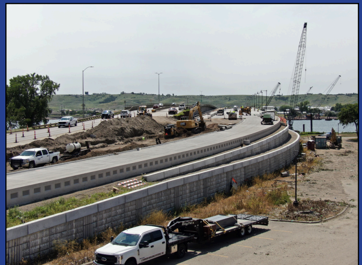
Exterior view of Pierre side barrier rail and MSE wall, July 15, 2024.
