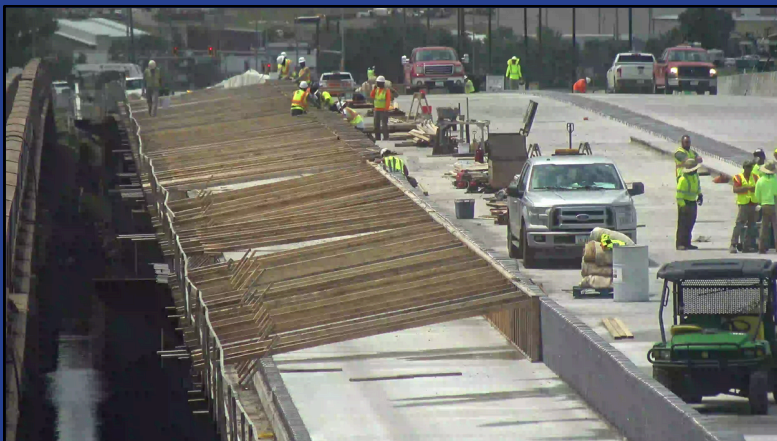
Separation rail in progress on the bridge deck, July 16, 2024.
