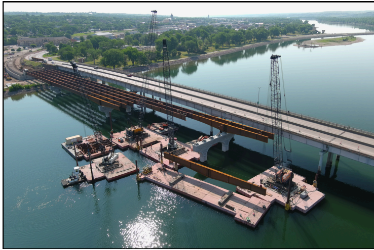
Girder installation on bent 4 and 5, June 12, 2023.
