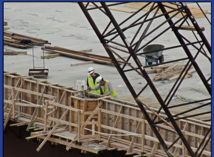
Workers take measurements in concrete forms for the upcoming barrier rail, June 17, 2024.
