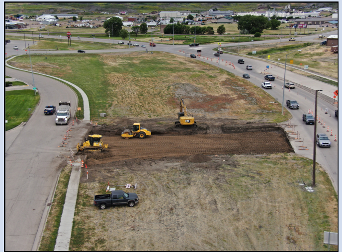
Earthmoving and grading for the Island Drive reconfiguration, June 17, 2024.
