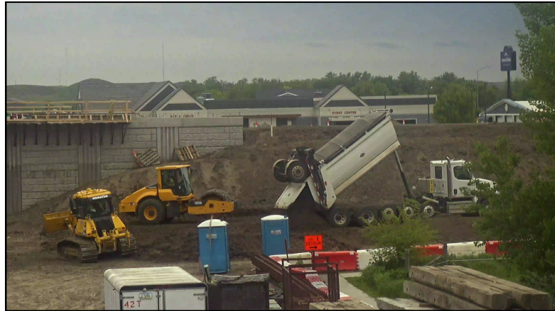
Installing additional earth for the end slope on the Ft. Pierre side, May 20, 2024.
