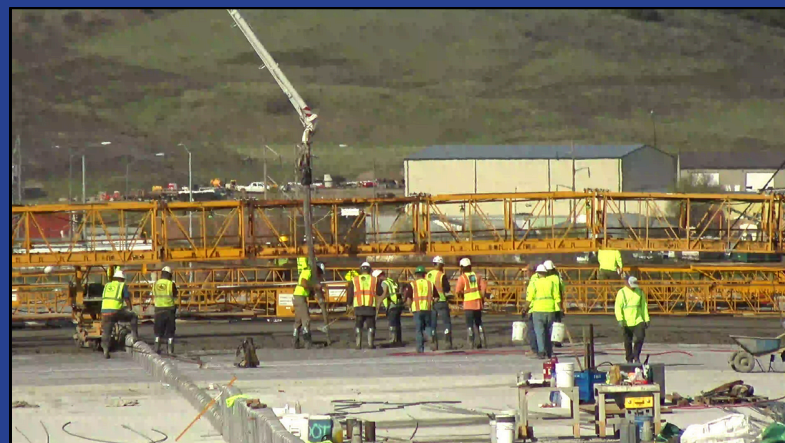
Workers pouring and paving concrete on the bridge deck, May 06, 2024.
