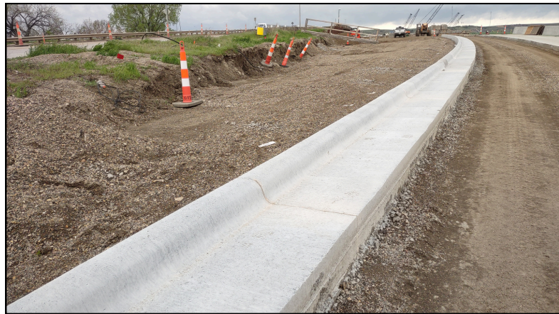
Curb strip placed on the Pierre side, May 06, 2024.
