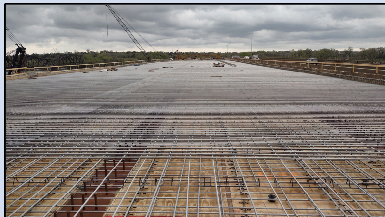
Steel rebar tied in and awaiting remaining concrete pours, May 06, 2024.
