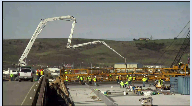
Extendable pump truck arm pouring concrete, May 01, 2024.
