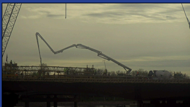
Extendable pump truck arm pouring concrete, May 03, 2024.
