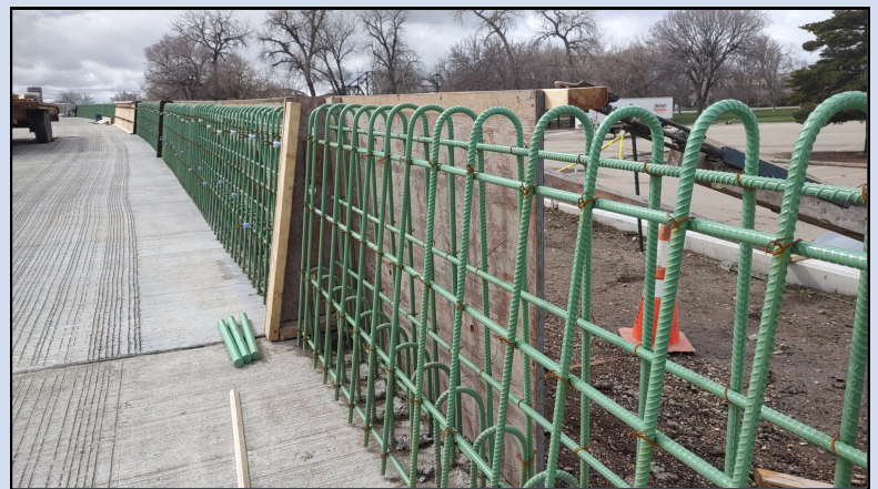
Epoxy-coated steel rebar in placement for barrier rail, April 08, 2024.
