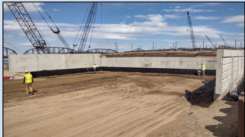
Workers packing earth for the upcoming Ft. Pierre abutment approach, March 19, 2024.
