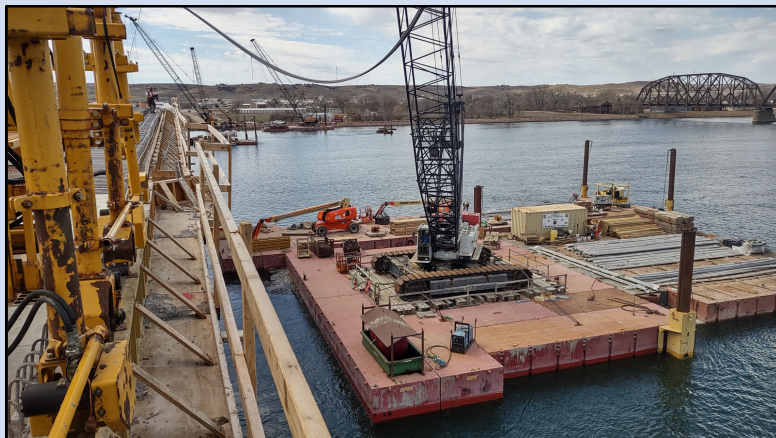
A barge crane delivers a load of rebar onto the bridge deck, March 19, 2024.
