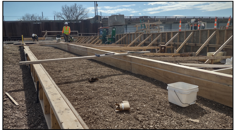
Concrete forms in place for sleeper slab, March 19, 2024.
