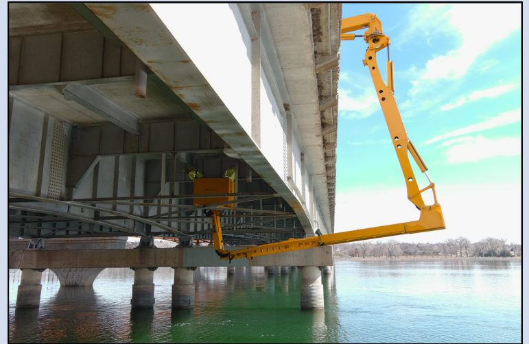
Workers on articulated boom lift inspecting the old bridge, March 11, 2024.
