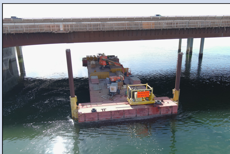
Transport barge with hydraulic stabilizers used as work area, March 11, 2024.
