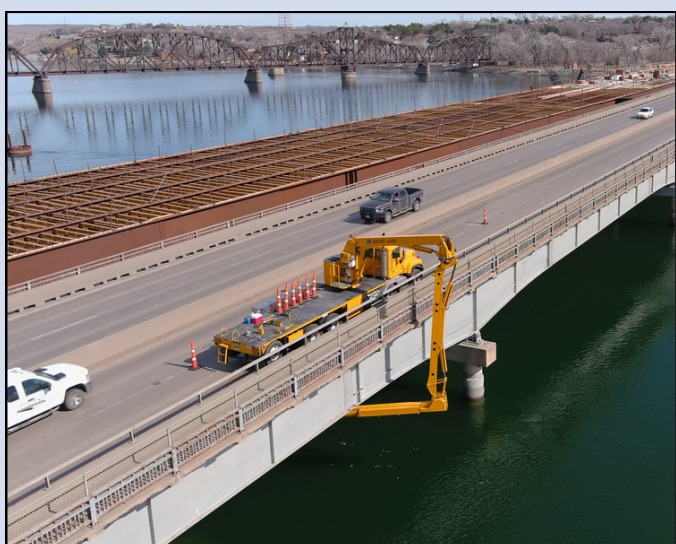
Workers on articulated boom lift inspecting the old bridge, March 11, 2024.
