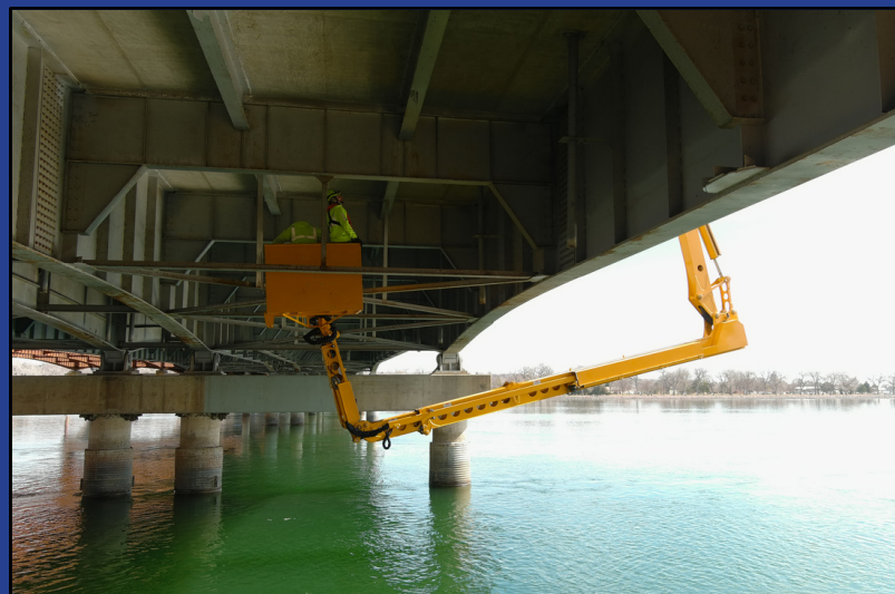
Workers on articulated boom lift inspecting the old bridge, March 11, 2024.
