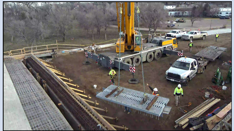
Mobile crane operator moving finger joint to the top of the east abutment, Feb. 26, 2024.
