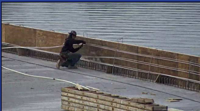
Worker installs rebar placement for upcoming barrier rail, Feb. 12, 2024.
