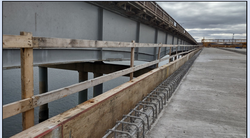
Wood forms and rebar placement in the pedestrian area on the downstream side, Feb. 13, 2024.
