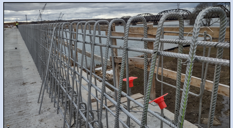
Rebar placement for the upstream side barrier rail, Feb. 13, 2024.
