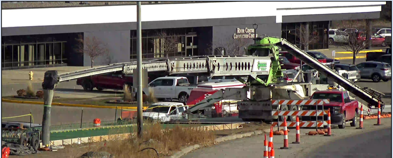
The telebelt is extended over the area of the planned moment slab, Dec. 5, 2023.
