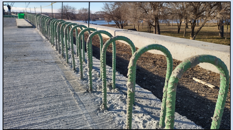
Steel reinforcement affixed within the concrete approach slab, Dec. 12, 2023.
