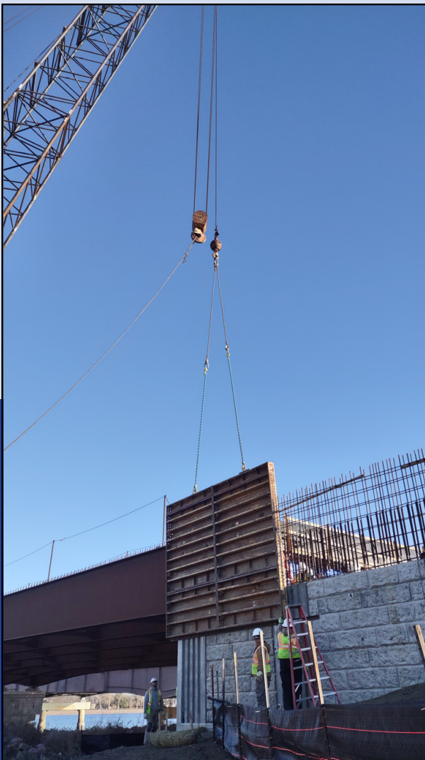
Workers guide an abutment form piece into place, Dec. 12, 2023.
