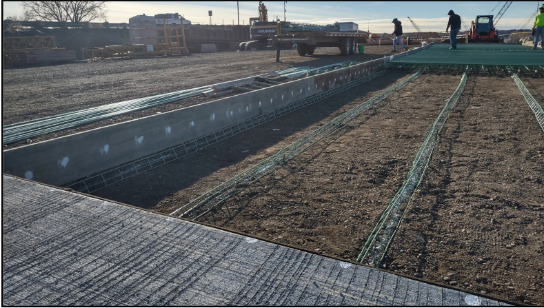
Prepping the next section of concrete approach slab, Dec. 12, 2023.
