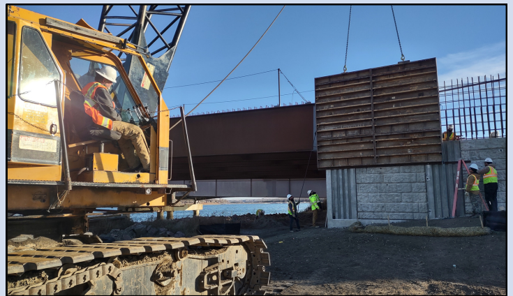
Placing abutment forms, Dec. 12, 2023.
